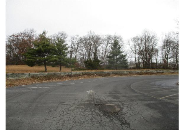
Sections of parking spaces can be converted to porous pavement to capture and infiltrate stormwater runoff from the parking lot. A preliminary soil assessment suggests that the soils have suitable drainage characteristics for green infrastructure.
