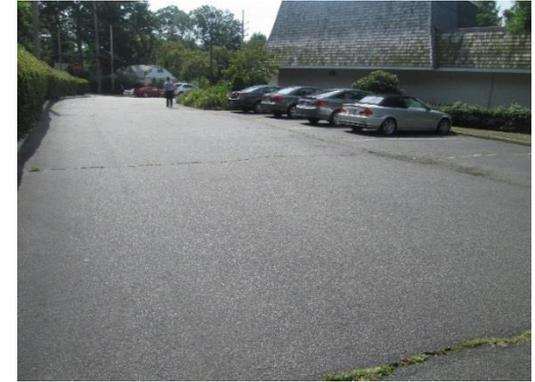
Runoff from the parking lot is directed to the stream behind the building. Parking spots can be replaced with porous asphalt to capture and infiltrate stormwater. The installation of a rain garden adjacent to the building can capture, treat, and infiltrate roof runoff. A preliminary soil assessment suggests that the soils have suitable drainage characteristics for green infrastructure.
