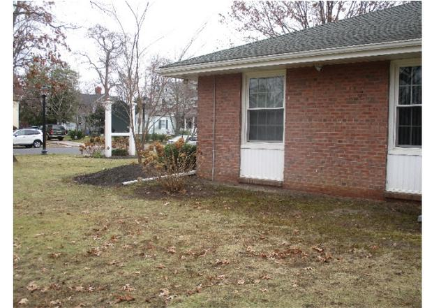
Rain gardens can be installed in the turfgrass area surrounding the building. The downspouts can be connected to the rain gardens so that they capture, treat, and infiltrate stormwater from the roof of the building. A preliminary soil assessment suggests that the soils have suitable drainage characteristics for green infrastructure.
