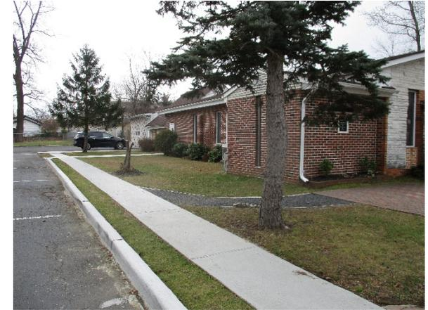
Rain gardens can be installed at three locations on the property to capture, treat, and infiltrate stormwater runoff from the parking lot and roof. A preliminary soil assessment suggests that the soils have suitable drainage characteristics for green infrastructure.
