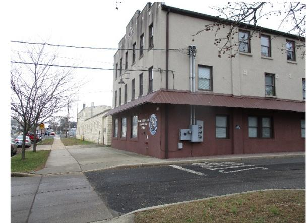
A section of sidewalk can be converted to a stormwater planter to capture, treat, and infiltrate stormwater runoff from the Board of Education's building roof and sidewalk. A preliminary soil assessment suggests that more soil testing would be required before determining the soil's suitability for green infrastructure.
